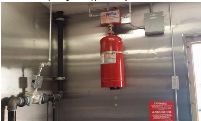
Inspecting Commercial Hood System
