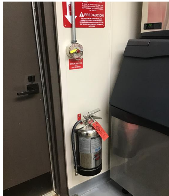
Inspecting Fire Safety Equipment
