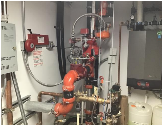
Inspecting Fire Suppression Systems
