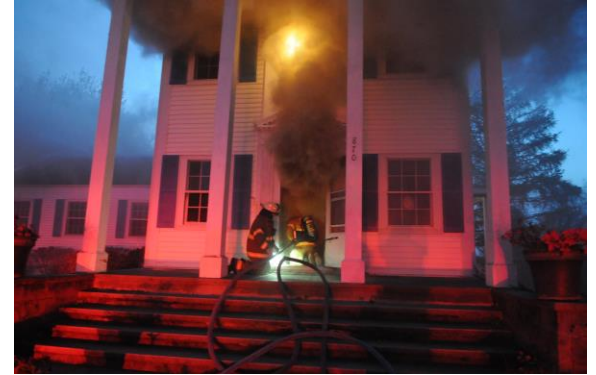
Structure Fire, Casco Twp
