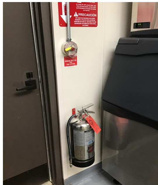
Inspecting Fire Safety Equipment
