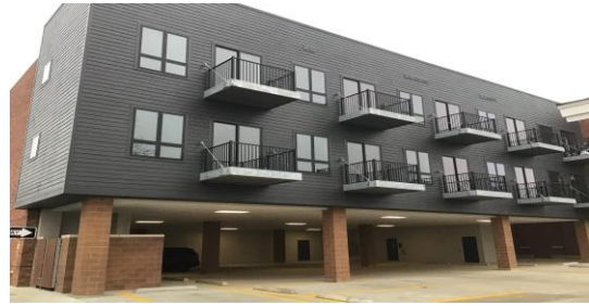
Inspecting New Construction
