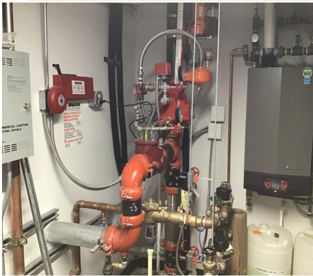
Inspecting Fire Suppression Systems
