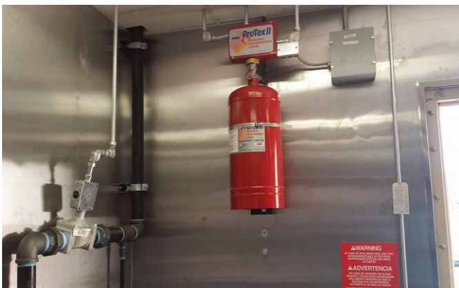
Inspecting Commercial Hood System
