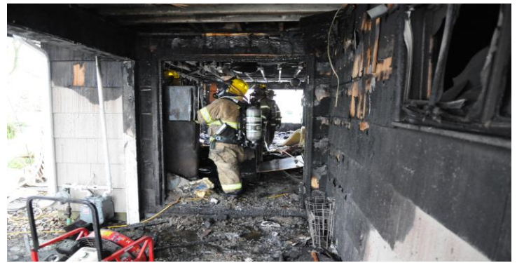
Structure Fire City of South Haven
