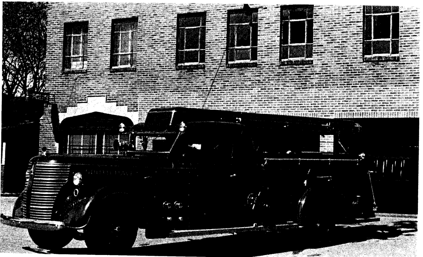
This 1946 model American LaFrance had a 12-cylinder engine capable of pumping 1,000 gallons of water per minute. It remained in service more than a quarter of a century.
