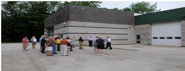
New addition to station #3 completed
