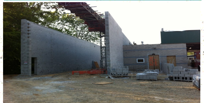
New addition to SHAES Station #3
