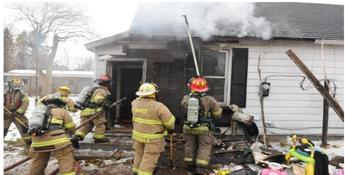
Structure Fire Geneva Twp
